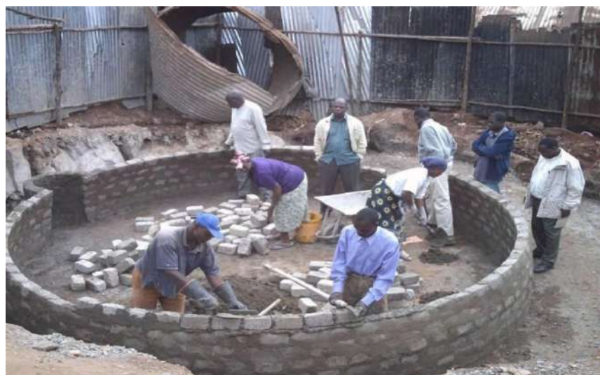
Fig No. 5.11: Biogas Digester under construction.
